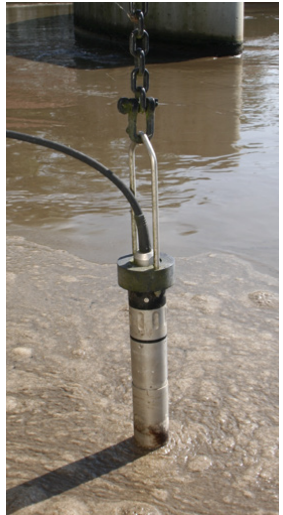
YSI IQ SensorNet ISE probe installed in anoxic zone of biological tank
